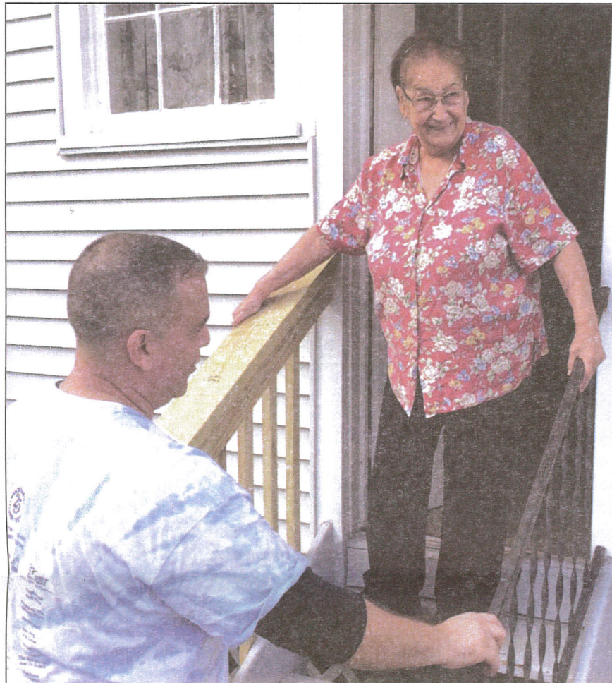
A homeowner admiring her new stair railing.
